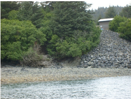
Photo 5: Riprap below Port Graham school gymnasium and erosion area. 2007
